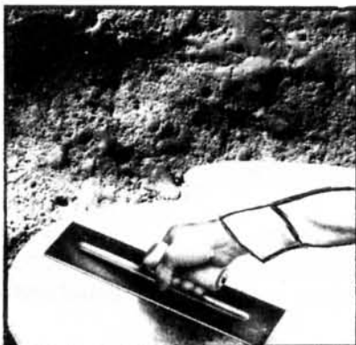
PLAS-TEX topping may be troweled as thin and smooth as desired.
